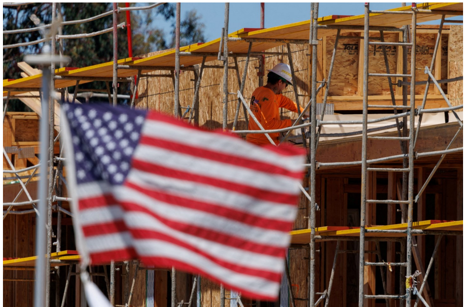
A construction worker is shown at work on a multi-unit residential housing project in Encinitas, California, July 28, 2025. REUTERS/Mike Blake
